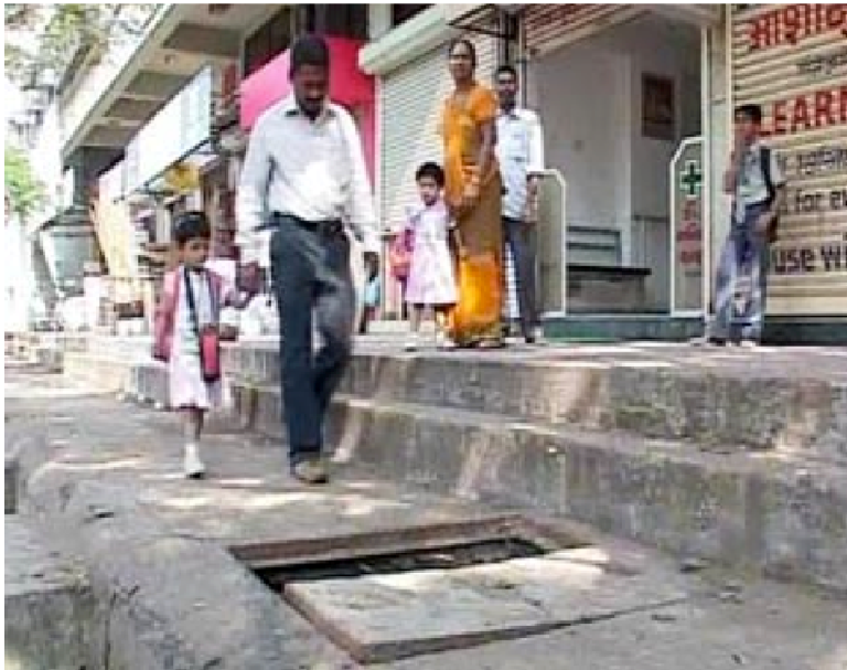
Picture 1: Uncovered manholes on pedestrian walk spaces in India
